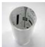
sample of pipe inspection
